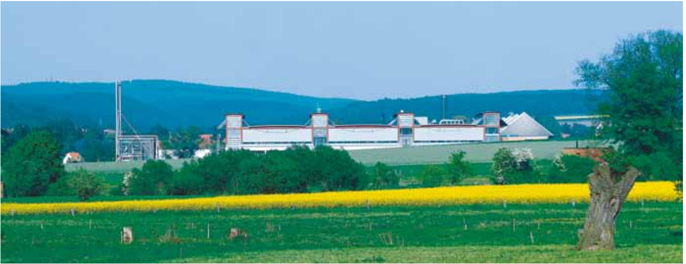
Back in 1996, the German Environmental Foundation presented Wilkhahn with an award for its impressive concept. The ecological and socially responsible management style is reflected in the architecture of the plant.
