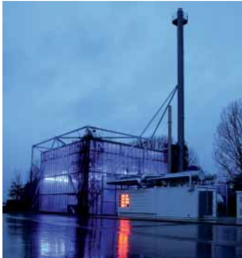
Co-generator powered by renewable raw materials
